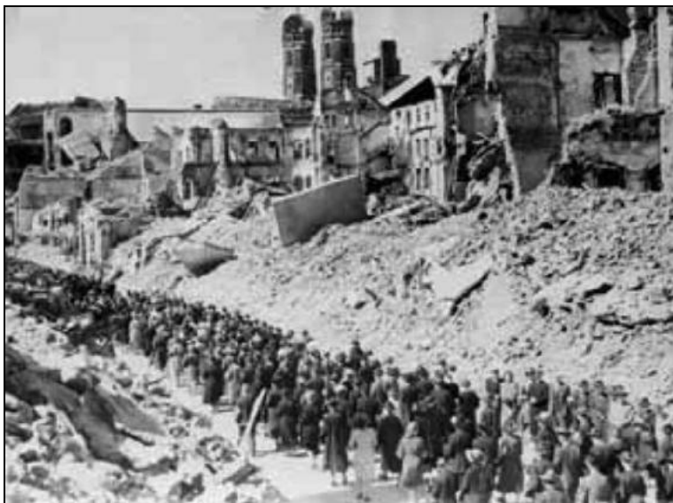
Munich on May 31, 1945, destroyed by the Allies bombings, two months
